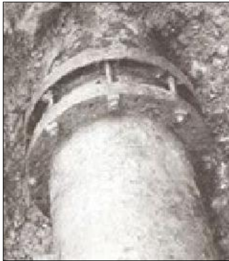
1953 Dresser coupling found in New York's Allegheny State Park in excellent condition after 50 years of service.
