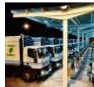
Compressed Natural Gas Dispensing
